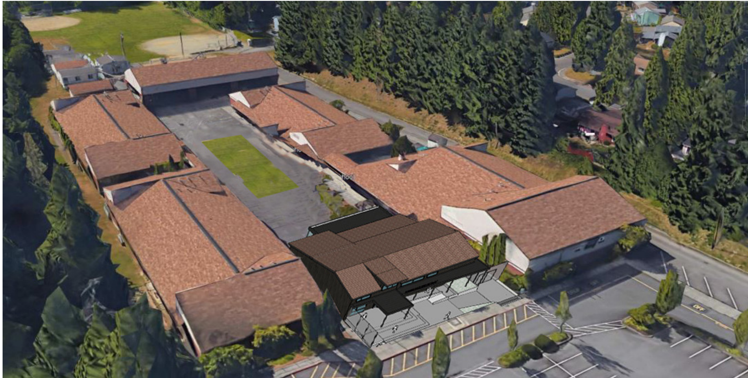
AERIAL VIEW - AFTER
